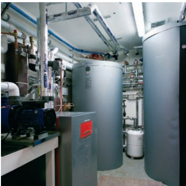
Below The thermal storage unit is linked to roof-mounted solar thermal panels and a ground source heat pump. The store supplies domestic hot water and the underfloor heating. Biomass heating provides as a secondary heat source to the main living spaces. The plant room also accommodates an MVHR (heat recovery) unit which extracts warm air from bathrooms and the kitchen, mixes it with fresh air and re-circulates it to the bedrooms.
